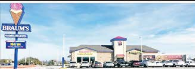
BRAUM'S IN ANADARKO is scheduled to re-open Monday, Nov. 13, the company announced today. The new store includes a Fresh Market, room for about 65 diners and a modern exterior. The former Braum's was torn down five months ago after being in operation for 33 years at that location.
